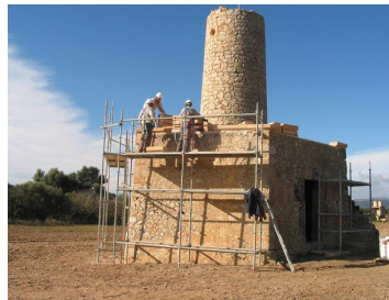
Restoration work at a former wind mill
